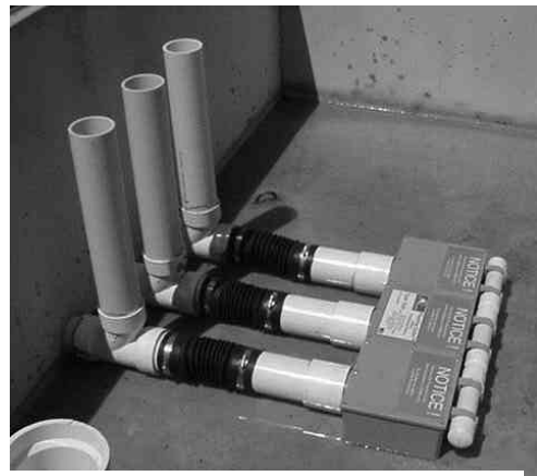
Figure 3. Three units joined and extended for increased draw-down and even dosing to three trenches of a large leachfield system.
